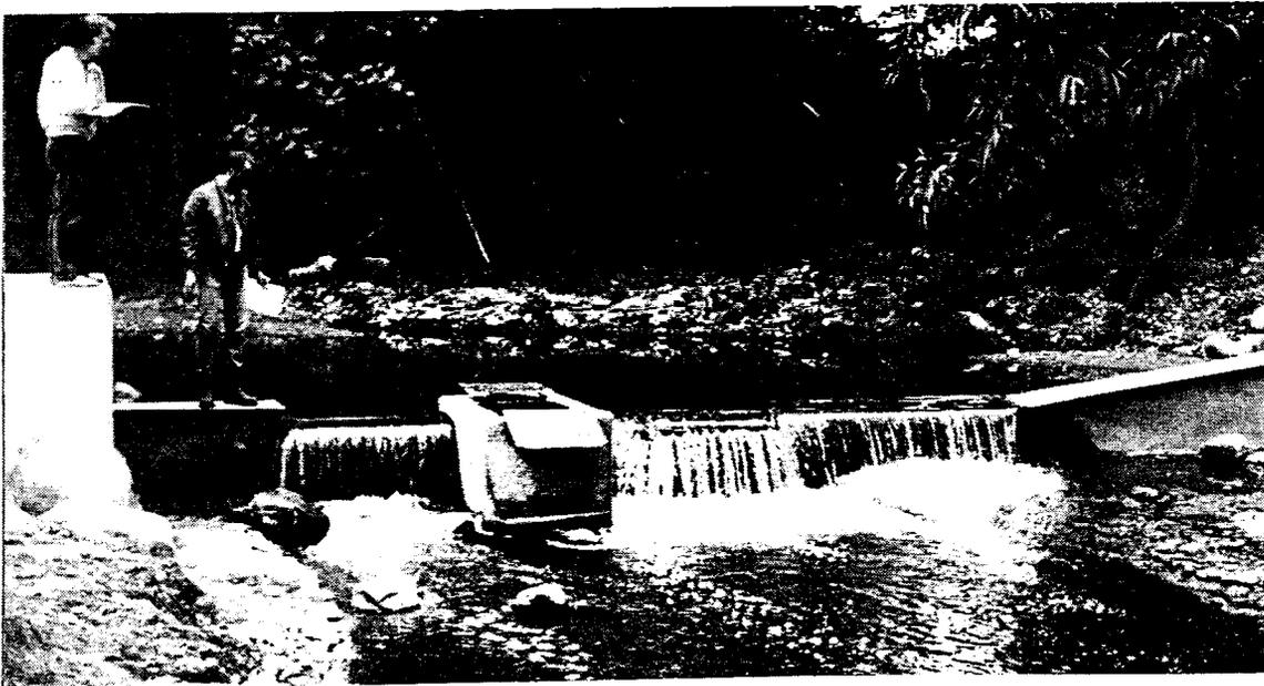
2. Sea lamprey barrier dam on Lakeport Cre& Lake Ontario, Ontario. It is a low head lamprey barrier dam with a built-in lamprey trap constructed in 1984.
