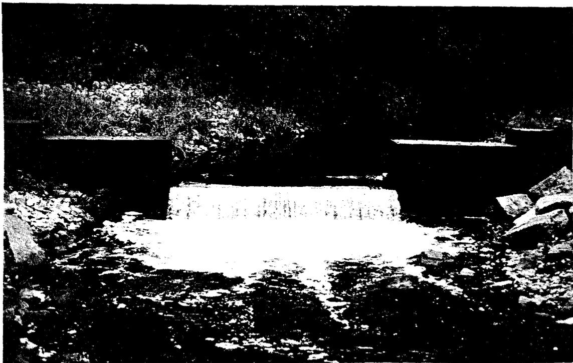
9. Sea lamprey barrier dam on the Sturgeon River, Lake Huron, Ontario. It is one of the earlier low headbarrier dams constructed in 1979 with steel sheet piling. It has a fish pass gate and jumping pool for passing jumping salmonids, but no lamprey trap.
