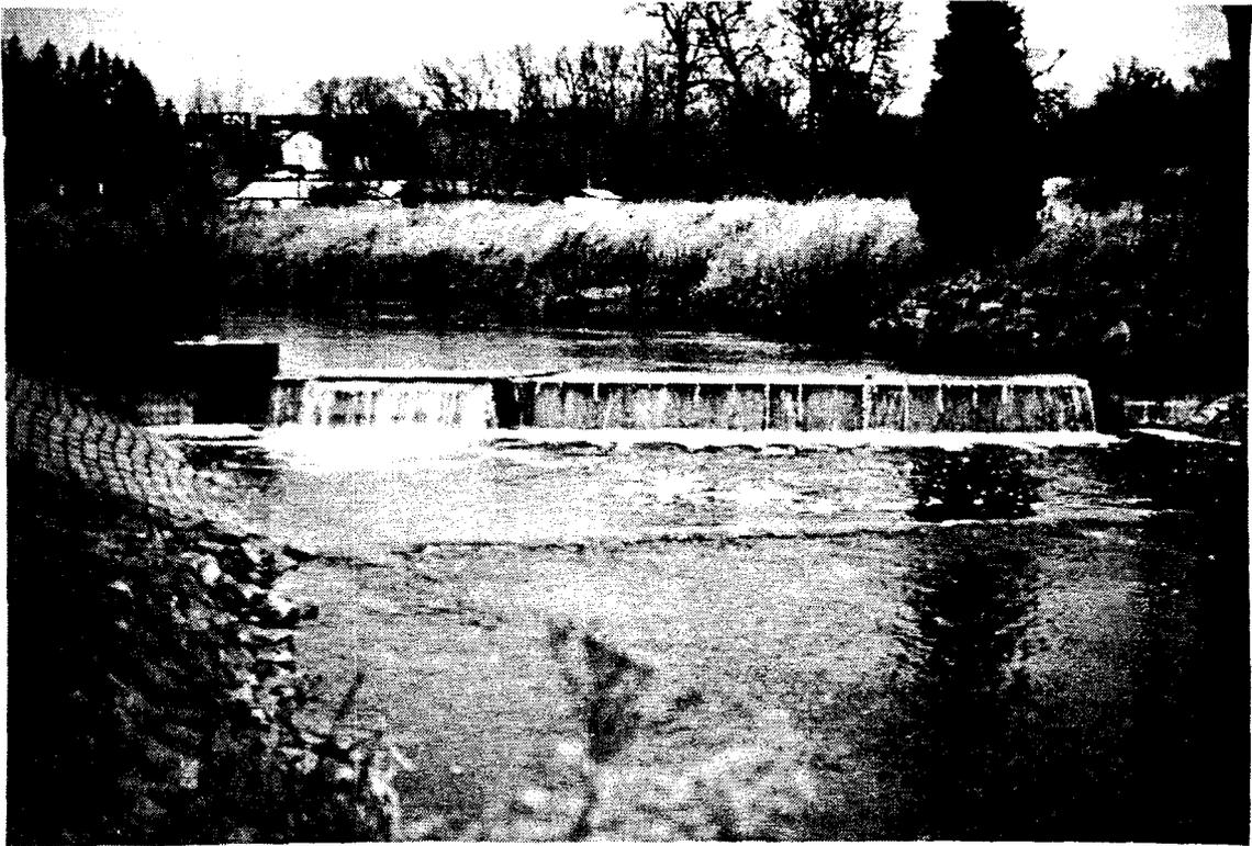
4. Sea lamprey barrier dam on Graham Creek, Lake Ontario, Ontario. It is a low head barrier dam constructed of steel sheet piling in 1983 and has a built-in lamprey trap and jumping pool.
