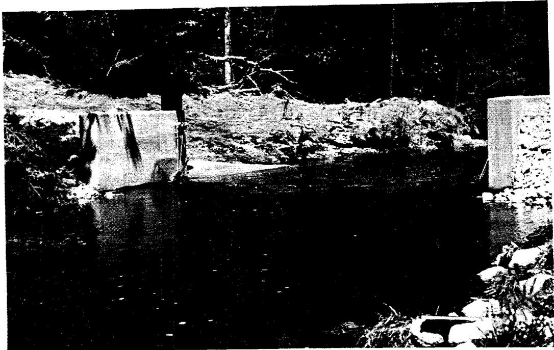
22b. Barrier dam on Albany Creek in July with gate lowered to allow for fish passage.
