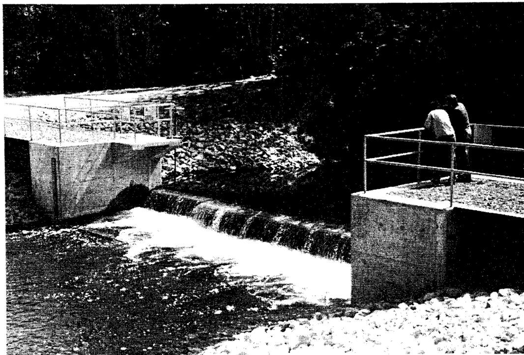
27. Sea lamprey barrier dam on the Misery River, Lake Superior, Michigan. A low head barrier dam constructed of concrete in 1984 with a slidegate to permit drawdown. It has a jumping pool and portable assessment traps.
