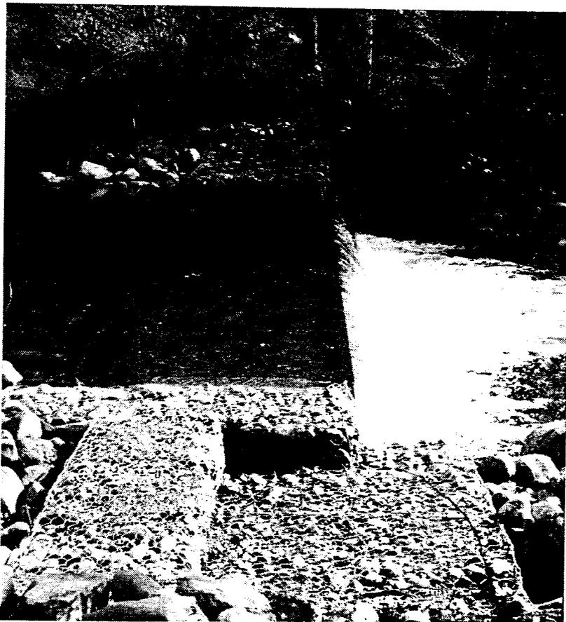
16. Sea lamprey barrier dam on Sheppard Creek, Lake Superior, Ontario. It is a low head barrier dam constructed in 1984 with gabions and has a jumping pool, but no lamprey trap.
