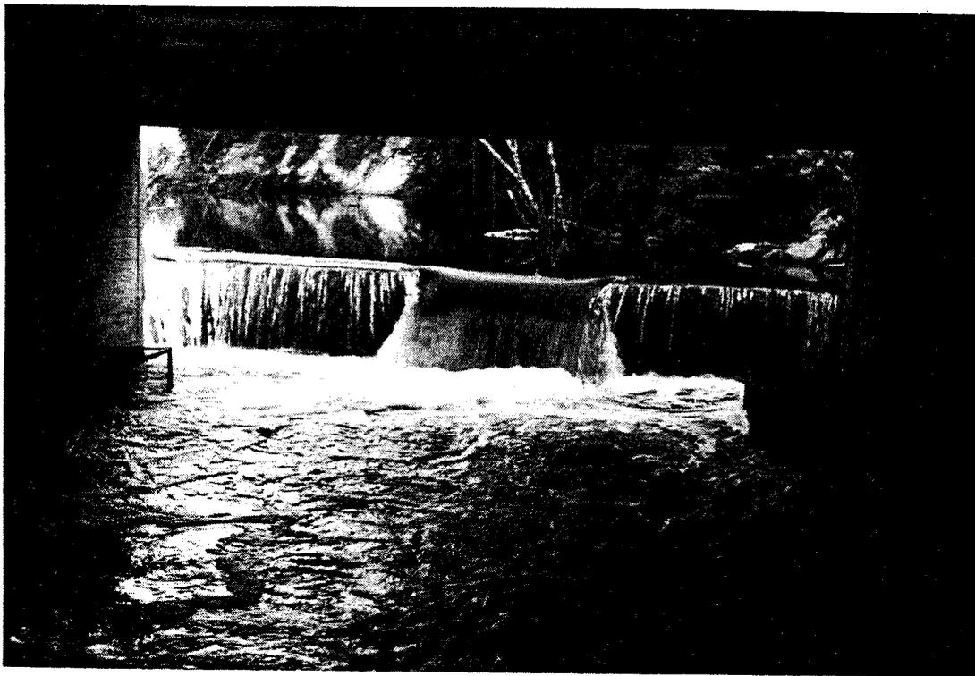
26. Sea lamprey barrier dam on Miner's River, Lake Superior, Michigan. A  $> 1$  m head concrete dam constructed in 1978 with stop logs to permit drawdown. It has a jumping pool and portable assessment traps.
