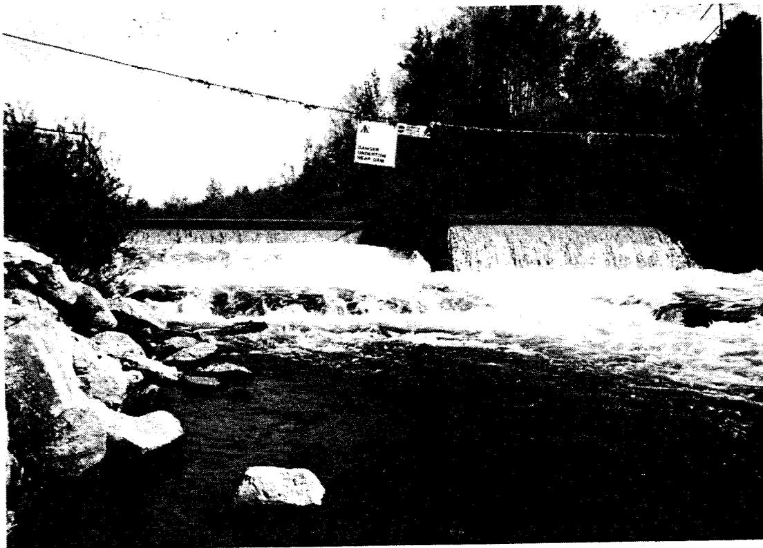
23. Sea lamprey barrier dam on the Betsie River, Lake Michigan, Michigan. An old hydra-electric dam was replaced in 1974 using **Anadromous Fish Conservation Funds**. It is a steel sheet piling structure, 1.8 m high (6 ft) and has a jumping pool.
