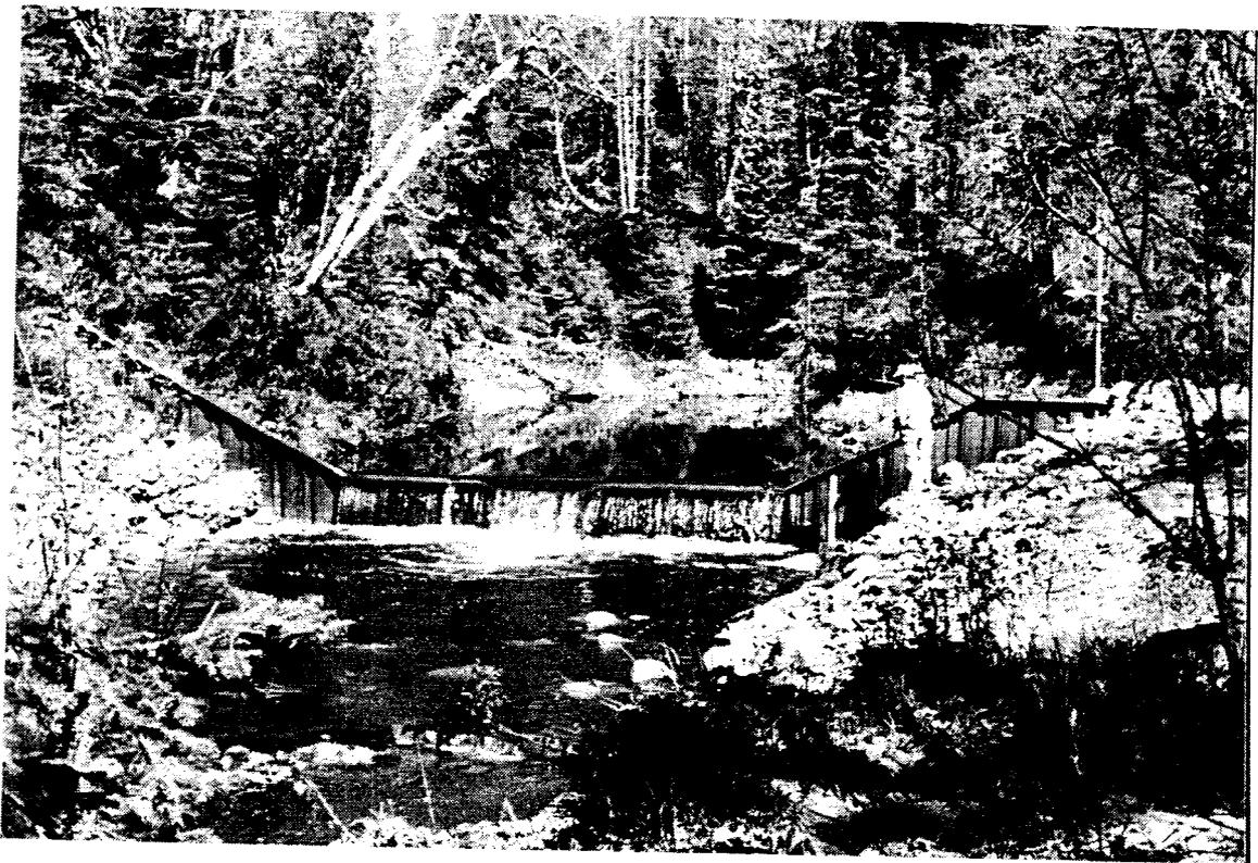
19. Sea lamprey barrier dam on Gimlet Creek, Lake Superior, Ontario. It is one of the earlier low head barrier dams constructed in 1979-80 of steel sheet piling and has a jumping pool, but mtatrap for lamprey.
