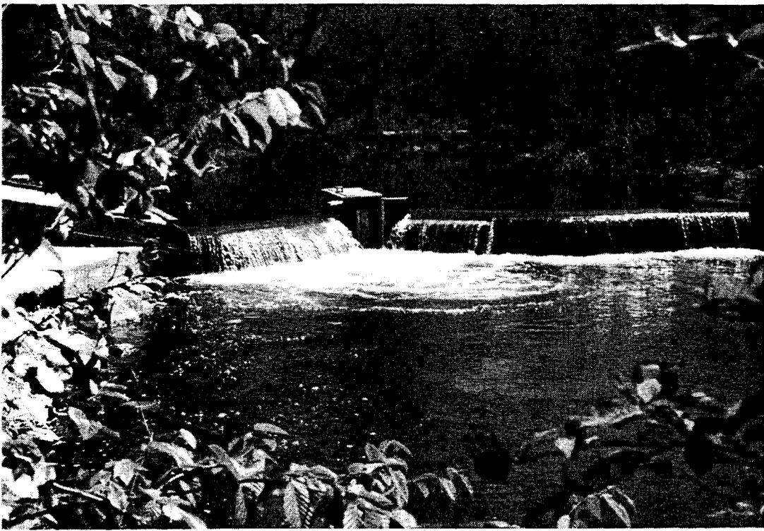
17. Sea lamprey barrier dam on Stokely Creek, Lake Superior, Ontario. A low head barrier dam constructed with steel sheet piling in 1980. It has a built-in lamprey trap and jumping pool.
