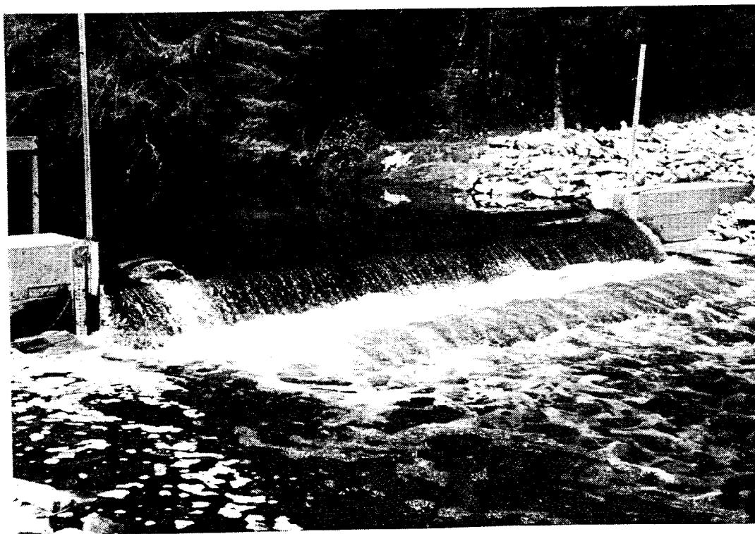
24. Sea lamprey barrier dam on Days River, Lake Michigan, Michigan. A concrete low head barrier dam constructed in 1983 with a lift gate to permit drawdown. It has a jumping pool and portable assessment traps.
