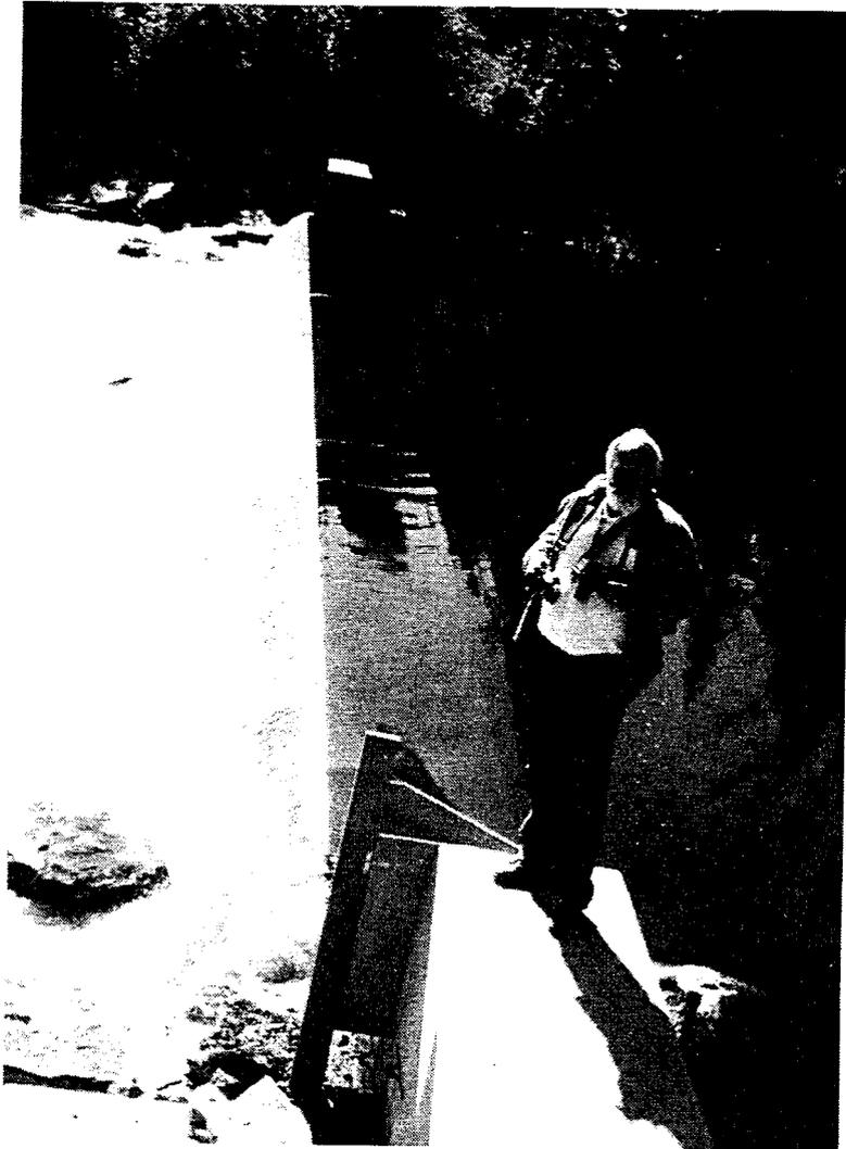
25. Sea lamprey barrier dam on West Branch of Whitefish River, Lake Michigan, Michigan. A low head concrete dam constructed in 1980. It has a permanent crest, jumping pool and portable assessment traps.
